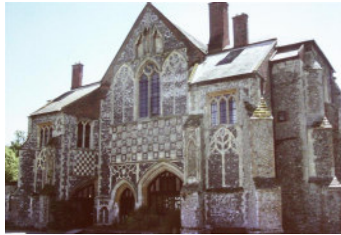
Butley Priory—some fine examples of flintworking techniques
